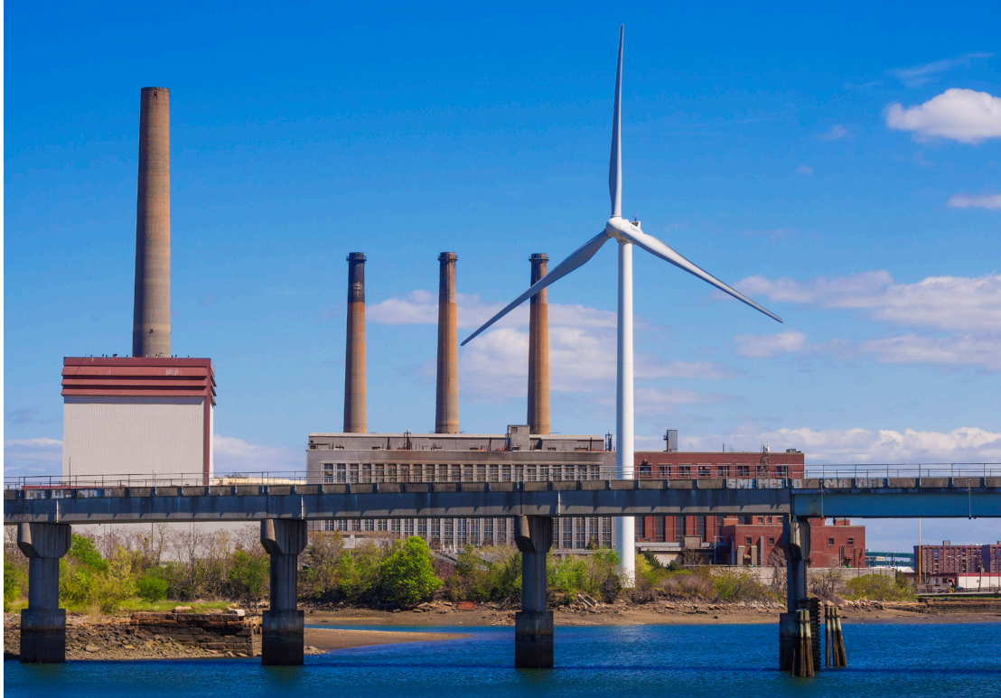
Wind turbine at the Massachusetts Water Resources Authority (MWRA) pump station by the Mystic River, Boston, MA. Source: Maudib/iStock/Getty Images Plus
